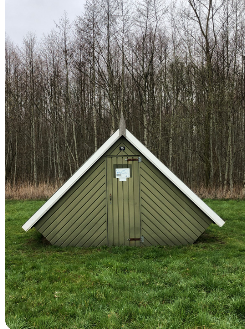
A salt hut at the cavern in the east of the Netherlands. Salt huts serve to protect the pipelines coming up from the ground.
