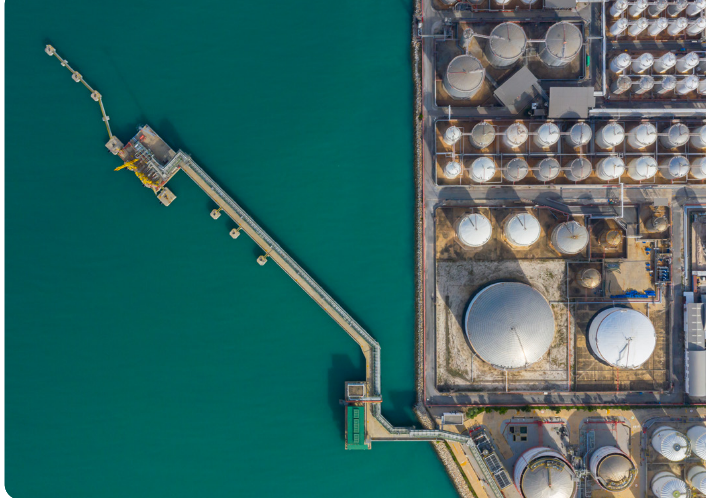
Oil terminal with landing jetty
