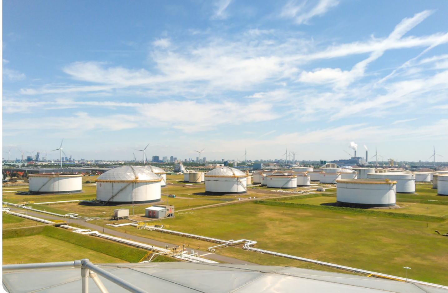
Tanks terminal in the north of the Netherlands (Image Ministry of Economic Affairs and Climate Policy)
